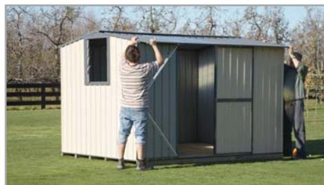
**Step 1: Boxed sheds only.** Unpack and read the instructions. Have your tools on hand. Join the sheets to form the wall panels and fix channels to top and bottoms. Bear in mind your door is already assembled and pre-hinged by our team. Complete all panels as per instructions and have them ready to erect your shed.
